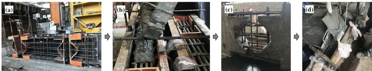
**Fig. 9** The production process of the specimens: **a** fabrication of formwork and reinforcement, **b** pouring pre-cast part UHPC, **c** joint splicing, and **d** pouring post-cast joint part UHPC
