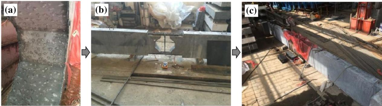
**Fig. 2** Manufacture process of test model: **a** roughening the surface, **b** splicing the pre-cast parts, and **c** natural curing the joint part
