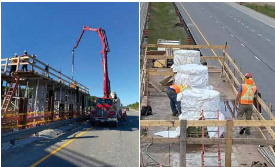
Fig. 1: Use of GFRP bars in bridge columns in Canada
