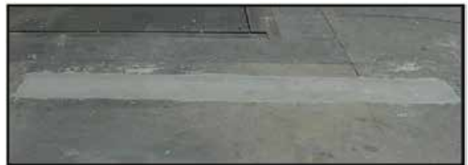
Fig. 2: Plumbing cutout after repair
