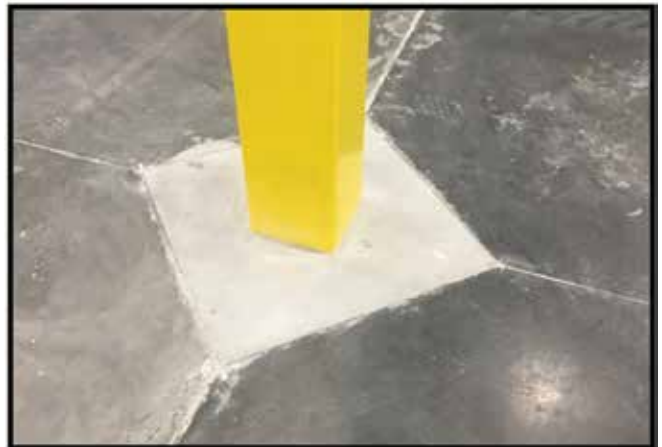
Fig. 3: Column blockout after repair
