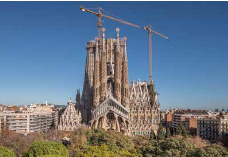
Fig. 2: The Passion façade features two 112 m (367 ft) bell towers flanked by two 102 m (334 ft) bell towers. Behind these, six more towers are under construction (© Fundació Junta Constructora del Temple de la Sagrada Família)
