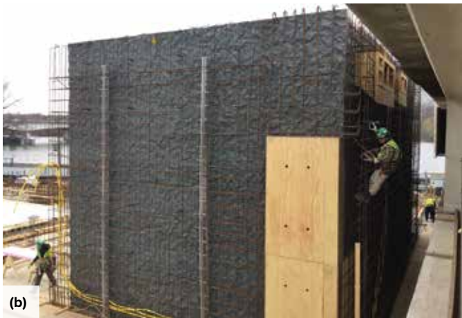
Fig. 14: Although interior walls were to be painted, the surfaces were complex and required very high attention to detail. To maintain a 5 x 4 ft (1.5 x 1.2 m) tie-hole pattern and enable efficient use of the crinkle concrete form liners, conventional Aluma stud forms were used rather than modular gang forms: (a) exterior formwork for Studio K; and (b) interior formwork and crinkle concrete form liners for the Justice Forum
