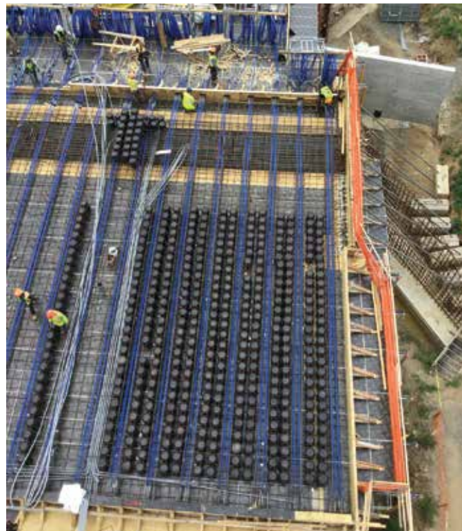
Fig. 2: A post-tensioned slab incorporating Cobiax void formers
