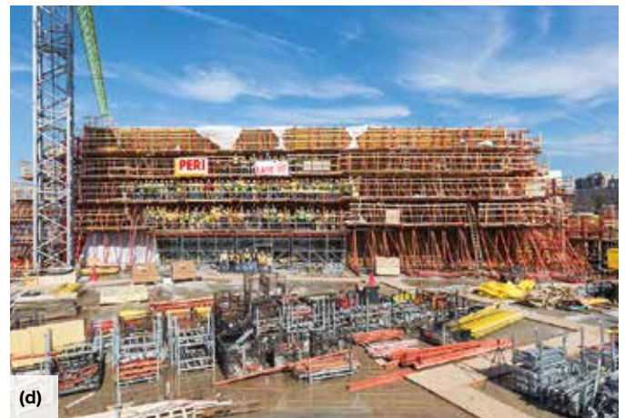
Fig. 9: The curved “feature” wall of the Skylight Pavilion required an extremely complex formwork system: (a) the initial formwork towers above the site, adjacent to the tower crane; (b) the tongue-and-groove board finish was especially challenging to create on the curved surface; (c) uniform tie spacing was required; and (d) the scale of the wall is made clear by this photo of the crew commemorating the final placement of the wall concrete
