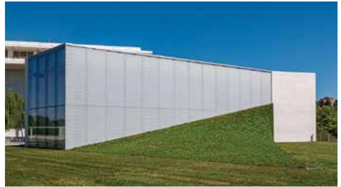
Fig. 4: The green roof near the Welcome Pavilion follows the contours of a vaulted ceiling in the pavilion below
