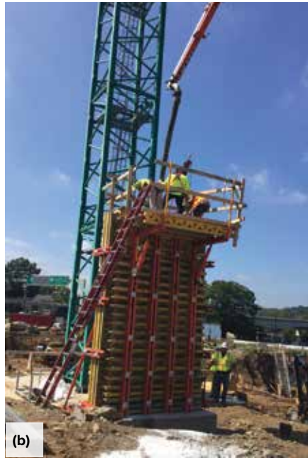
Fig. 16: Mockups were used to evaluate placement methods: (a) pumping at the base of the formwork; and (b) using the concrete pump hose as a drop chute
