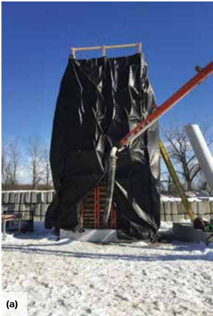
Fig. 16: Mockups were used to evaluate placement methods: (a) pumping at the base of the formwork; and (b) using the concrete pump hose as a drop chute
