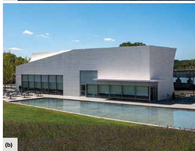
Fig. 10: A conical roof slab is a prominent feature of the River Pavilion. In contrast to the conical slab at the Welcome Pavilion, this feature was placed using a single layer of manually finished white concrete: (a) an interior view; and (b) an exterior view
