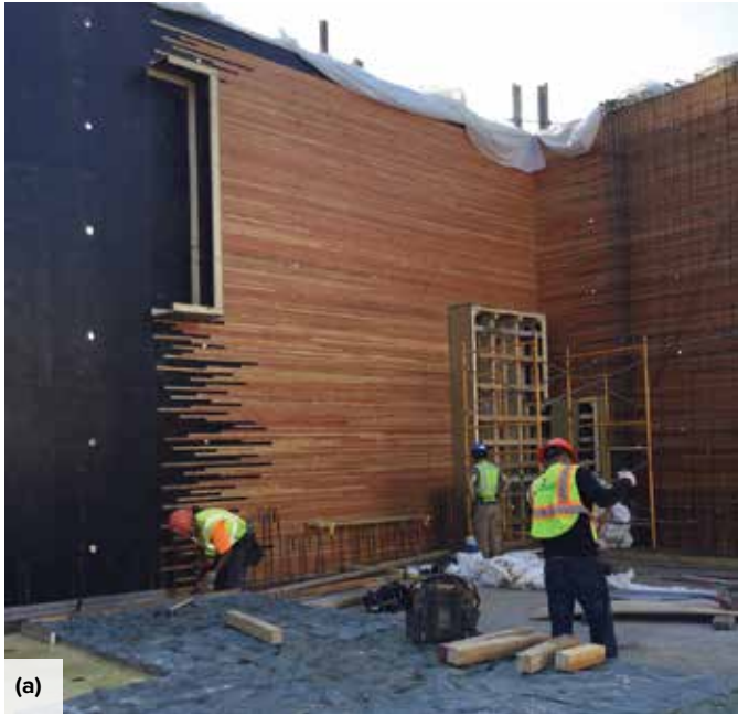
Fig. 15: Tall walls were fabricated with proprietary crack inducers to minimize the visual impact of contraction joints
