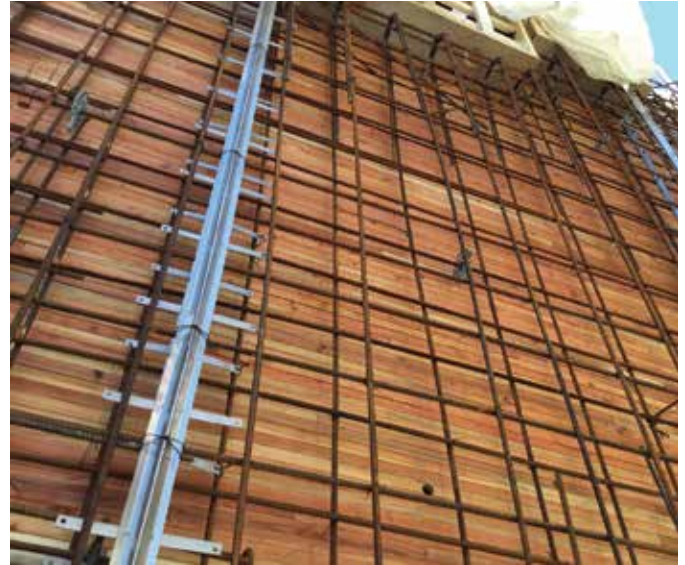
Fig. 15: Tall walls were fabricated with proprietary crack inducers to minimize the visual impact of contraction joints
