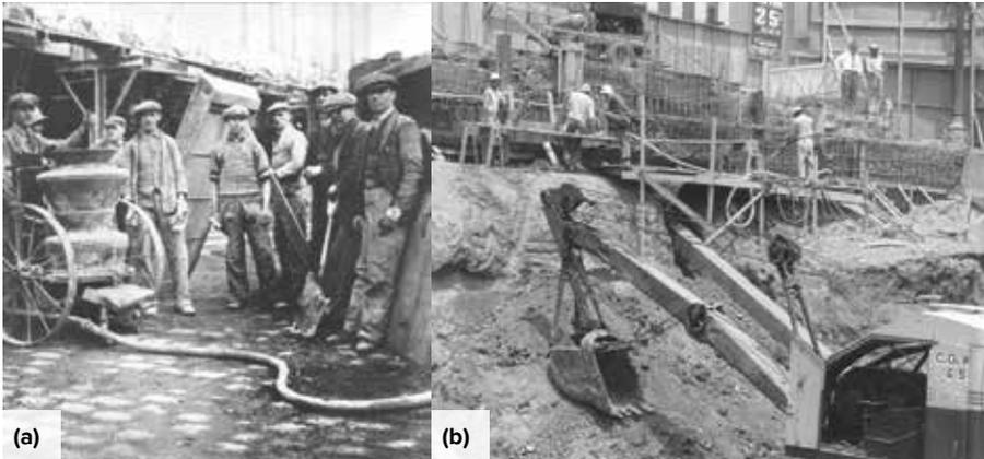
Shotcrete has been widely used for over a century: (a) a crew poses with their equipment in the 1920s; and (b) a crew places a foundation wall in the 1940s
