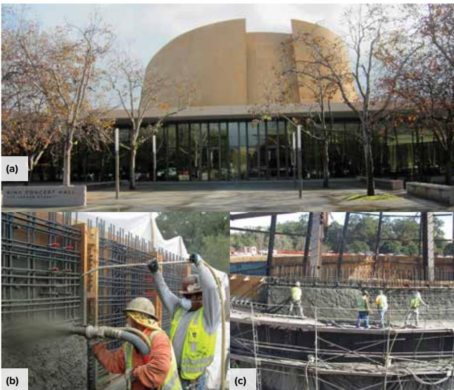
Shotcrete is ideal for placing complex structures: (a) the curved enclosure wall of Stanford University’s Bing Concert Hall comprises shotcrete with a sand float finish; (b) a certified nozzle operator and a blowpipe operator construct mockup panels for the enclosure wall; and (c) crews placed the 12 in. (300 mm) thick enclosure wall in multiple lifts, using a removable screed rail to control the thickness (photos courtesy of Joseph J. Albanese, Inc.)
