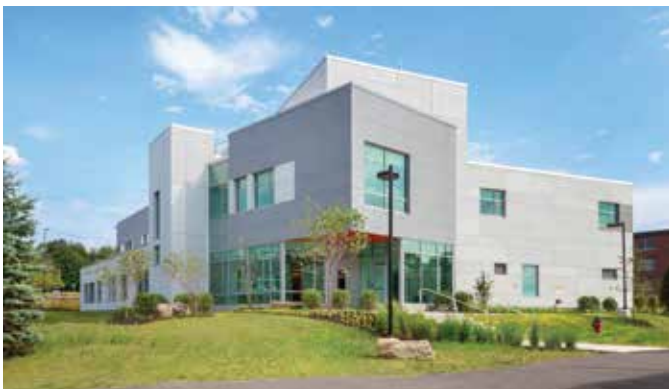
The new Engineering Innovation Hub's exterior walls feature HPC panels in light and dark gray (Photo courtesy of Ola Wilk/Wilk Marketing Communication)
