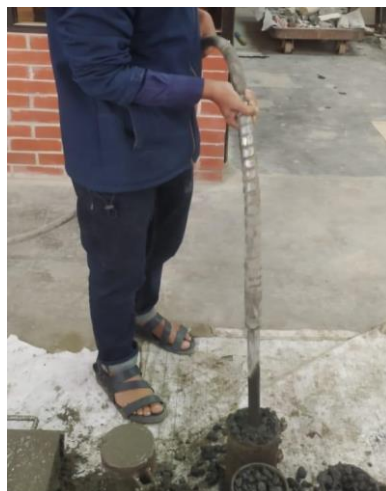
Fig 4.10: Compaction of concrete using vibrator
