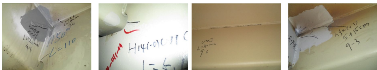
Fig. 1 Cracking condition after initial maintenance of the Junshan Yangtze River Bridge
