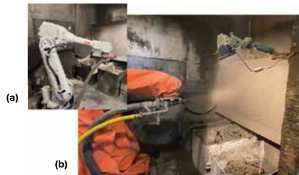
Fig. 1: ABB IRB-4600 Industrial Robot in the Shotcrete Laboratory at ULaval: (a) robot without its protective sleeve; and (b) robot spraying a large steel test panel (2 m wide x 1 m high [6.6 x 3.3 ft])
