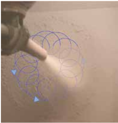
Fig. 2: Position of the center of the nozzle (solid line) and footprint of the material stream (green circle) during planetary motion spraying
