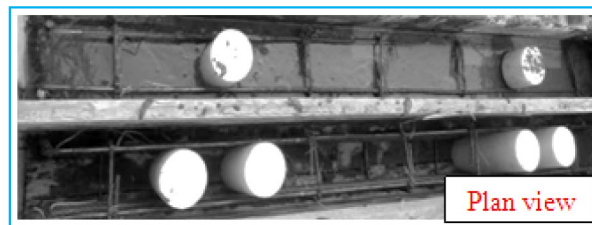
(b) Formworks after placing the reinforcing cage and during the casting
