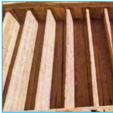
(a) Formworks before placing the reinforcing cage
