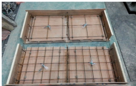
(a) Formworks and reinforcing bars
