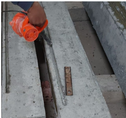
(b) Grooves were cleaned using a high-pressure air jet
