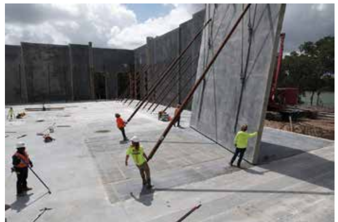
Euclid Chemical's EUCOTILT WB bond breaker used during tilt-up construction
