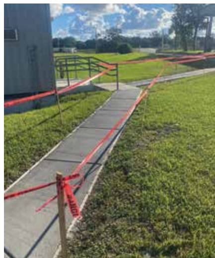
Fig. 3: Sidewalk with MSWI BA at the Solid Waste Authority of Palm Beach County, FL
