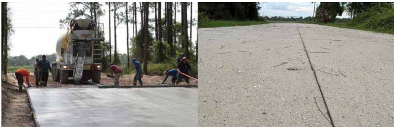
Fig. 4: Pasco County, FL, PCC section with MSWI BA coarse aggregate during construction (left) and a decade after (right)
