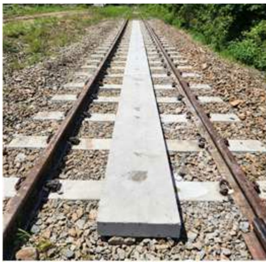
Fig. 5 Concrete panel-type DCP of ballasted track (DCP Type 1)
