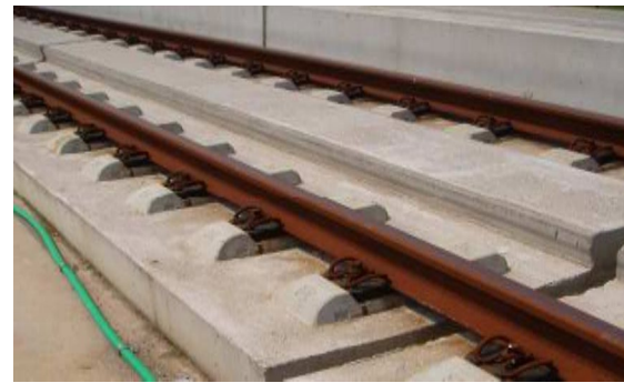
Fig. 3 Cast-in-place concrete plinth on Rheda concrete track (Hamilton & Inc, 2004)
