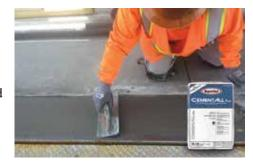
resistance for longer-lasting repairs in areas that experience significant temperature fluctuations. Cement All and Cement All Plus are both installed using traditional placement methods and can be floated or broom-finished in addition to troweled.
