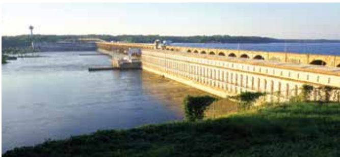
Internally cured concrete helped TVA meet resilience goals for the Wilson Dam (photo courtesy of United States Tennessee Valley Authority)
