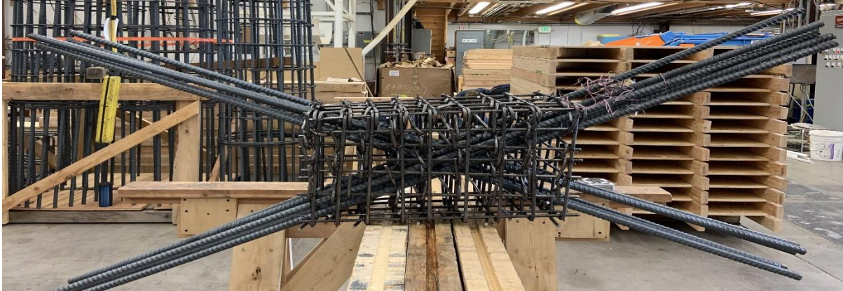
Figure 4.10. Reinforcement Cage for D(#6)-1.5-0.69
