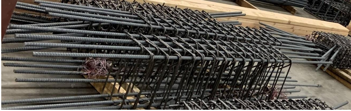
Figure 4.7. Reinforcement Cages for C(#5)-3.0-0.69 and C(#5)-3.0-0.35
