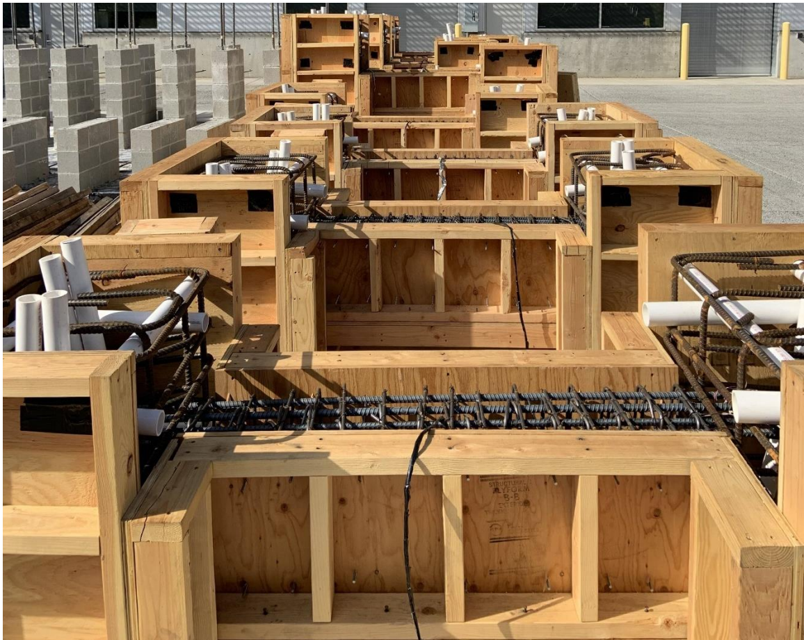
Figure 4.11. Reinforcement Cages in Formwork Prior to Pouring Concrete to Top of Beams
