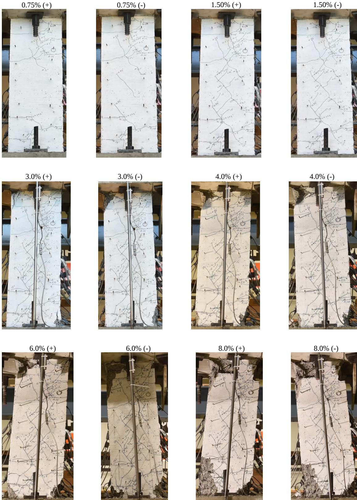
Figure 5.6. Damage Photos for D(#6)-3.0-1.38 at First Cycle Displacement Peaks
