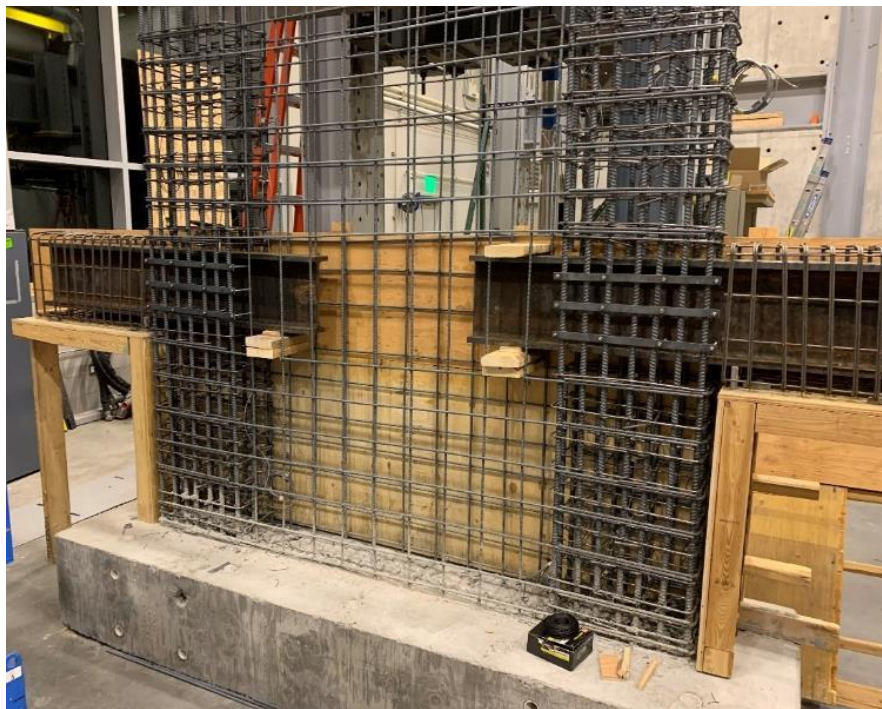
Figure 3.7. Photo of Reinforcement in Wall and Coupling Beams for SRC-W1 and SRC-W2
