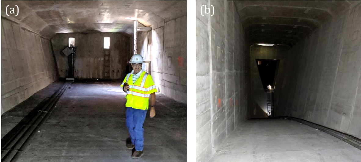
Figure 11: Inside SHSCB Showing the (a) End Diaphragm and (b) Pier Diaphragm
