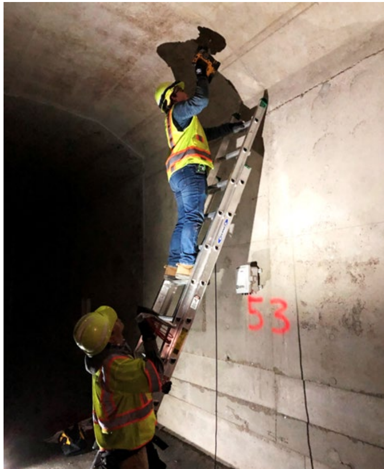
Figure 13: Installation of Strain Gauge in Section 1
