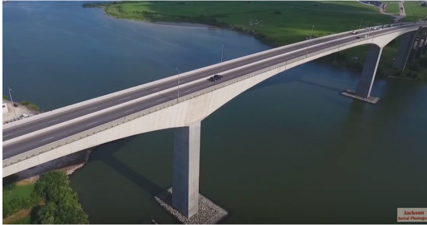
Figure 1: Sam Houston Ship Channel Bridge (SHSCB)
