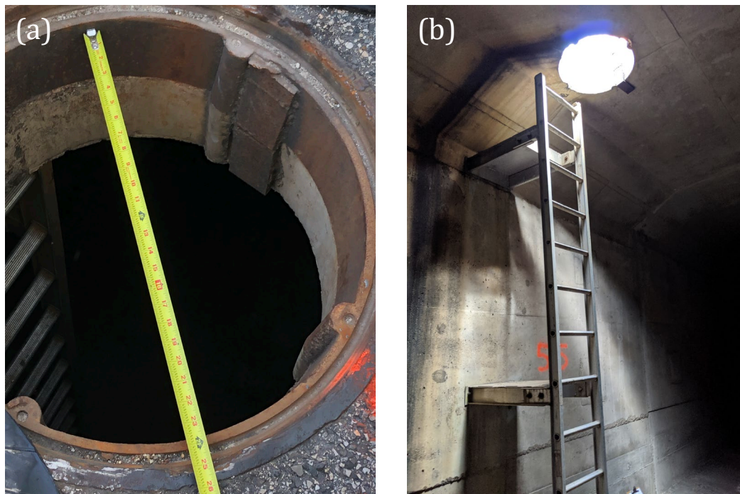
Figure 12: SHSCB (a) Manhole and (b) Ladder Access Inside the Segmental Box Girder
