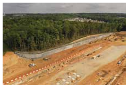
Aerial view of completed wall
