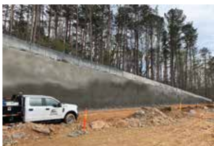
After shotcrete application that was placed by a robot
