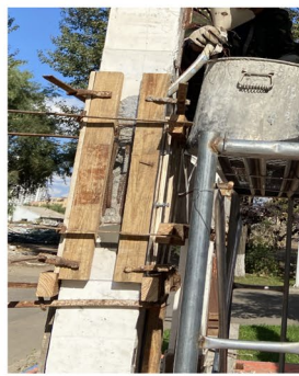
(c) Grout pouring
