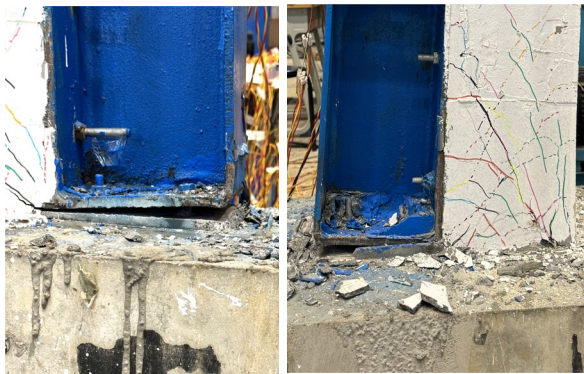
(a) Left column bottom, at negative loading (b) Right column bottom, at positive loading
