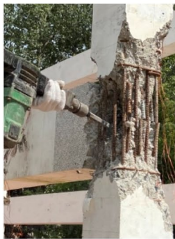
(b) Crushed concrete chipping
