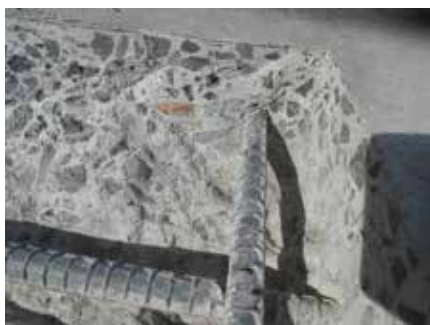
Fig. 3: Apparently well-bonded reinforcing steel without significant corrosion
