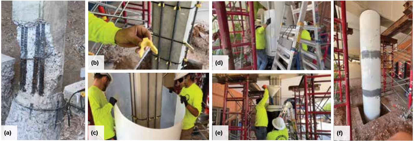
Fig. 1: Repair of a deteriorated column with a fiber-reinforced polymer (FRP) laminate: (a) damaged surface; (b) installing the spacers and reinforcing bars; (c) wrapping the first laminate to create a shell; (d) wrapping additional laminates; (e) filling the annular space; and (f) completed repair
