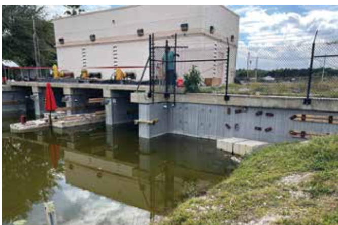
Fig. 5: Repair of corroded steel sheet piles in Weston, FL, USA, in June 2024
