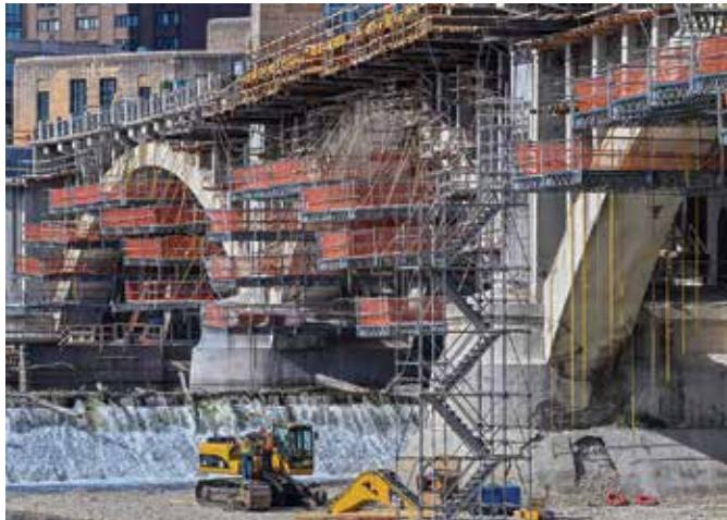
**Access to the substructure required complicated suspended scaffolding and dewatered cofferdams** (photo courtesy of Joe Szurszewski Photography)
