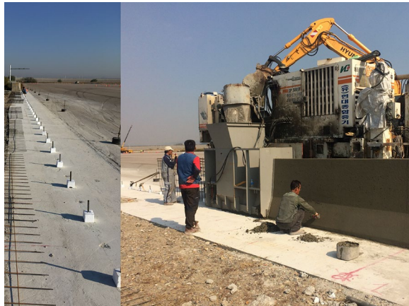
Fig. 16 Installation of the proposed CMB-17F: Styrofoam allows for deformation and slipforming of the concrete median barrier
