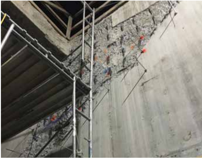
Fig. 7: Vertical patching repair
