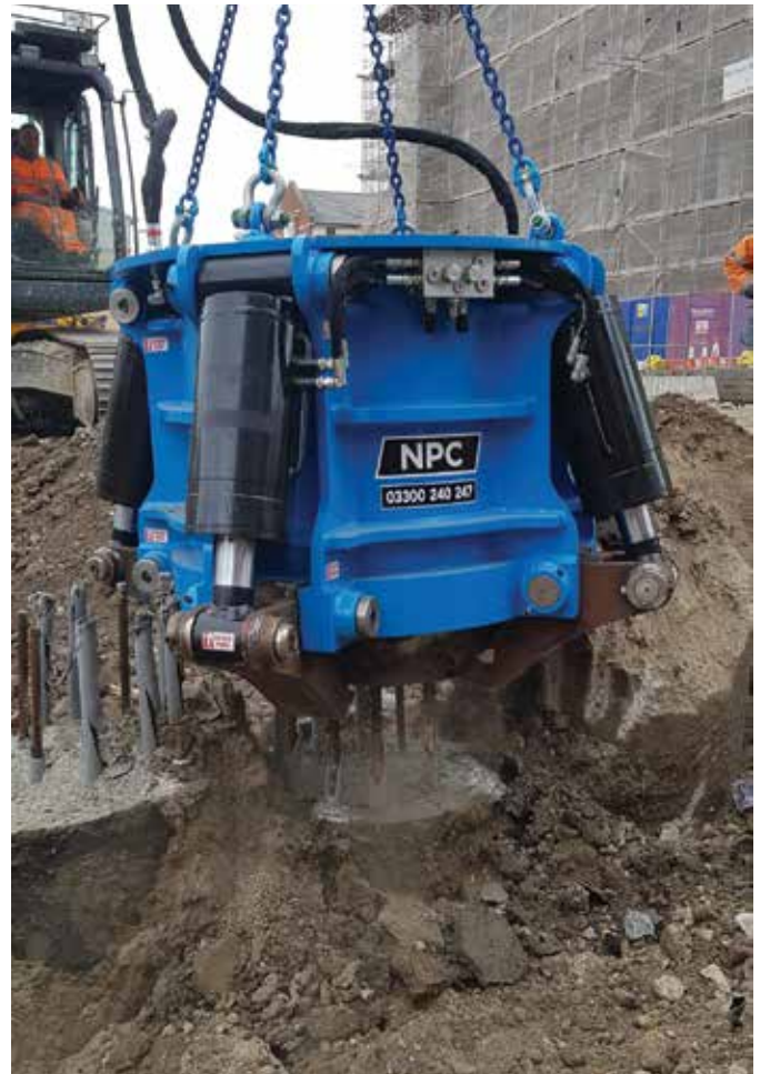
Fig. 1: A hydraulic pile cropper making a cut around reinforcing bars
