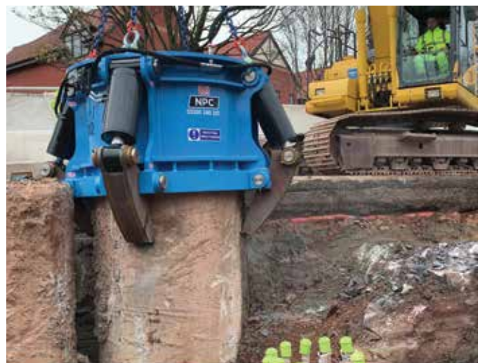
Fig. 2: The cropper positioned over the pile by the excavator lift
