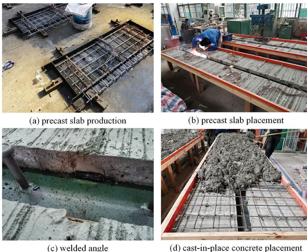
**Fig. 4** The fabrication process of the composite beam with precast slab: **a** precast slab production, **b** precast slab placement, **c** welded angle, **d** cast-in-place concrete placement.
