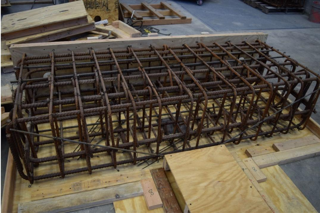
Figure B.5 – Base block reinforcement,
