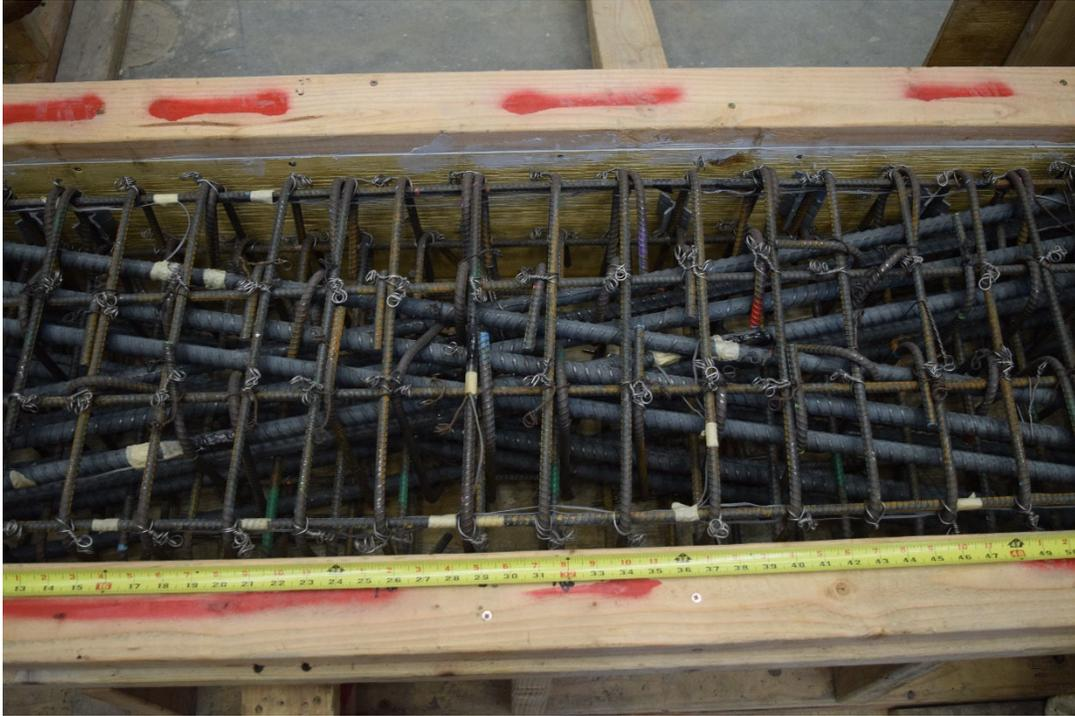
Figure B.3 – Coupling beam reinforcement, D120-3.5
