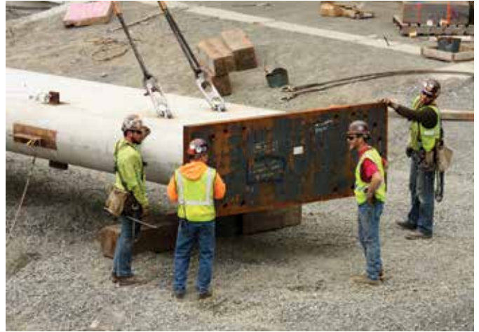
Shear-bolt couplers were welded to steel embed plates to connect longitudinal bars at the base of each wall
