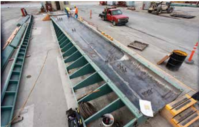
Workers are shown placing embeds in the steel form. After the reinforcing cage was installed, the top halves of the side forms were bolted in place to form the 180-degree radiused ends of the wall unit
