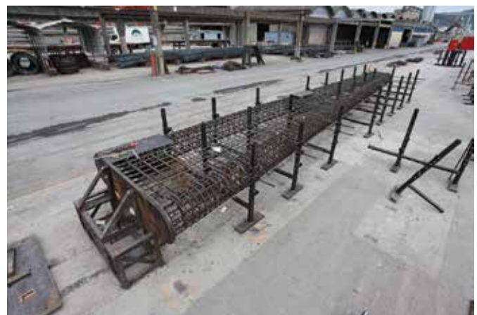
A typical concrete wall section and an assembled reinforcing cage
