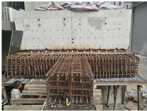
a Configuration of a wall-beam joint connected by welded steel plates
