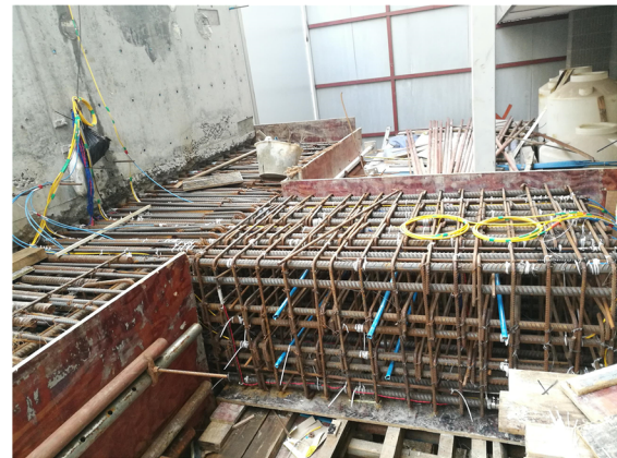
a Configuration of a wall-beam joint connected by mechanical couplers
