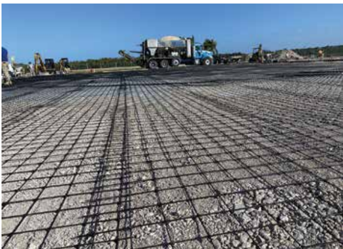
Fig. 5: FRP meshes can be used as secondary reinforcement in slabs-on-ground
