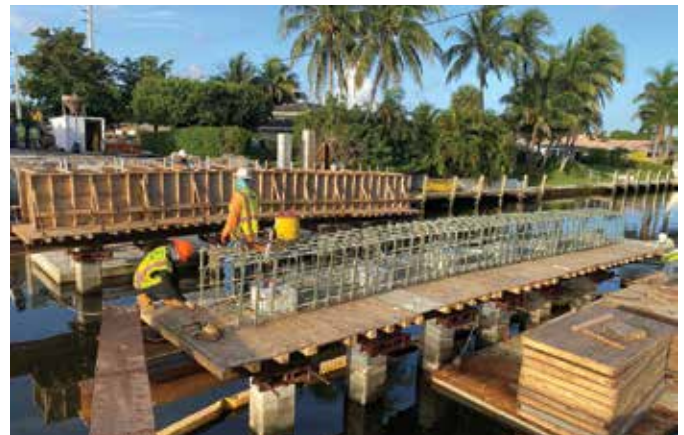
Fig. 4: A coastal bridge under construction. The piers and bent cap were reinforced with FRP reinforcing bars supplied in both straight and pre-bent forms
