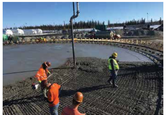
Fig. 6: Placing, vibrating, and finishing of concrete slab
