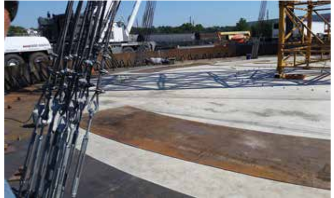
Fig. 7: Installation of skirt-sketch plate assembly prior to precast panel erection
