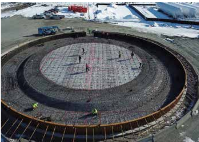
Fig. 3: View of floor-footing reinforcement
