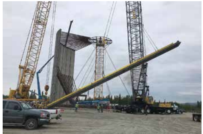
Fig. 9: Panel erection and bracing operations
