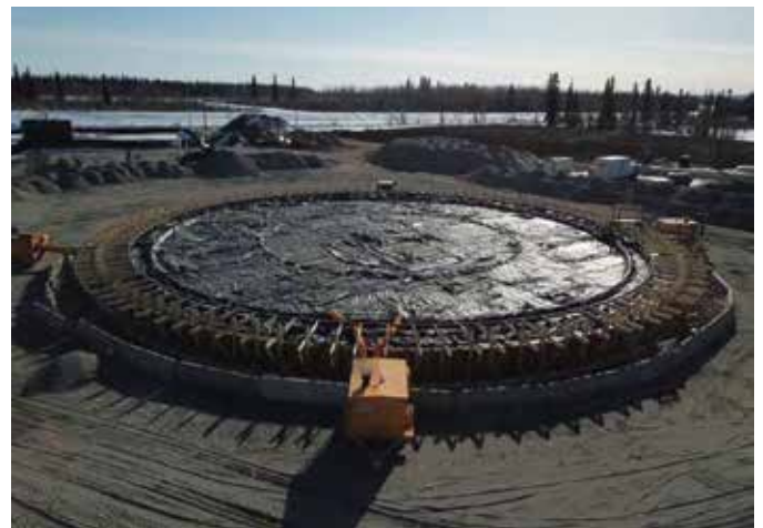
Fig. 4: Heating of reinforcement and top of subgrade 12 hours prior to placement
