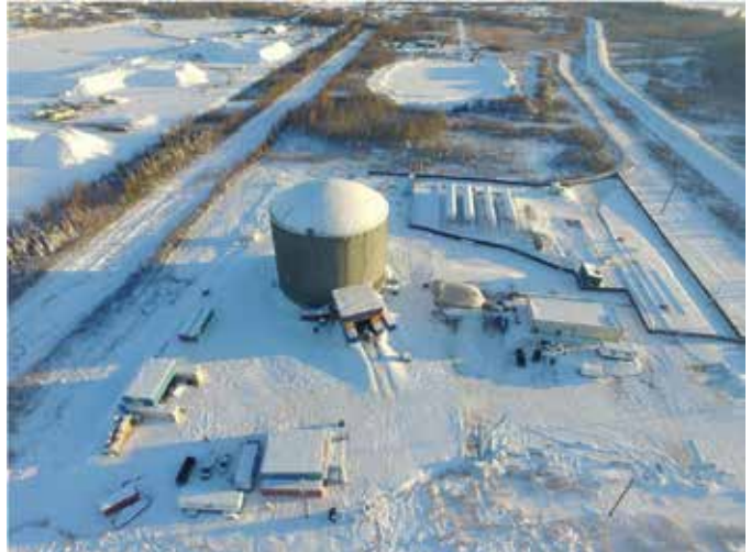
Fig. 11: View of outer concrete tank after completion of circumferential prestressing
