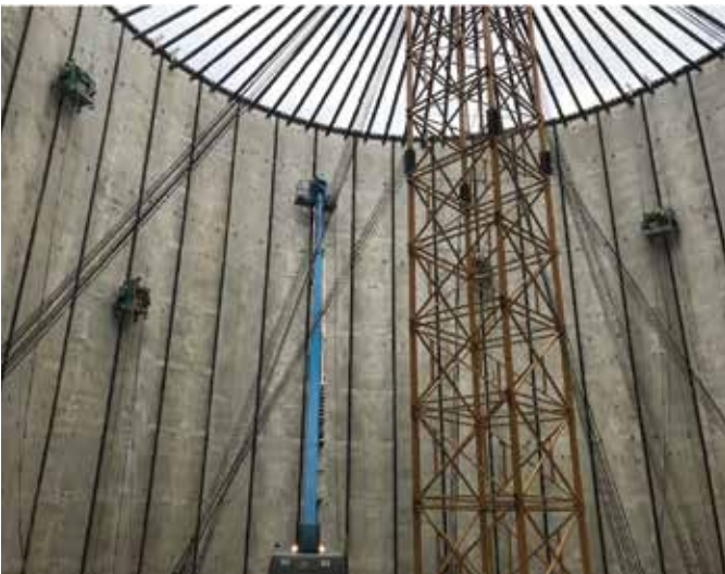
Fig. 10: Shotcreting of joints between precast panels
