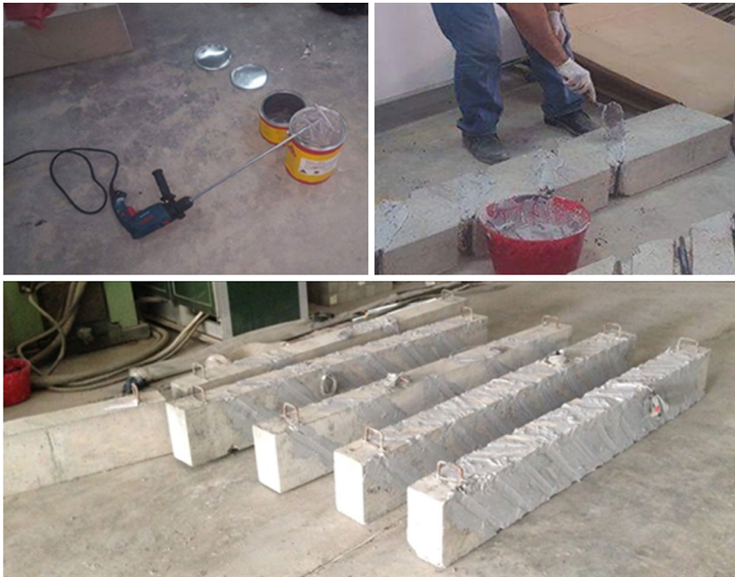
Fig. 5 Groove filling with epoxy.
