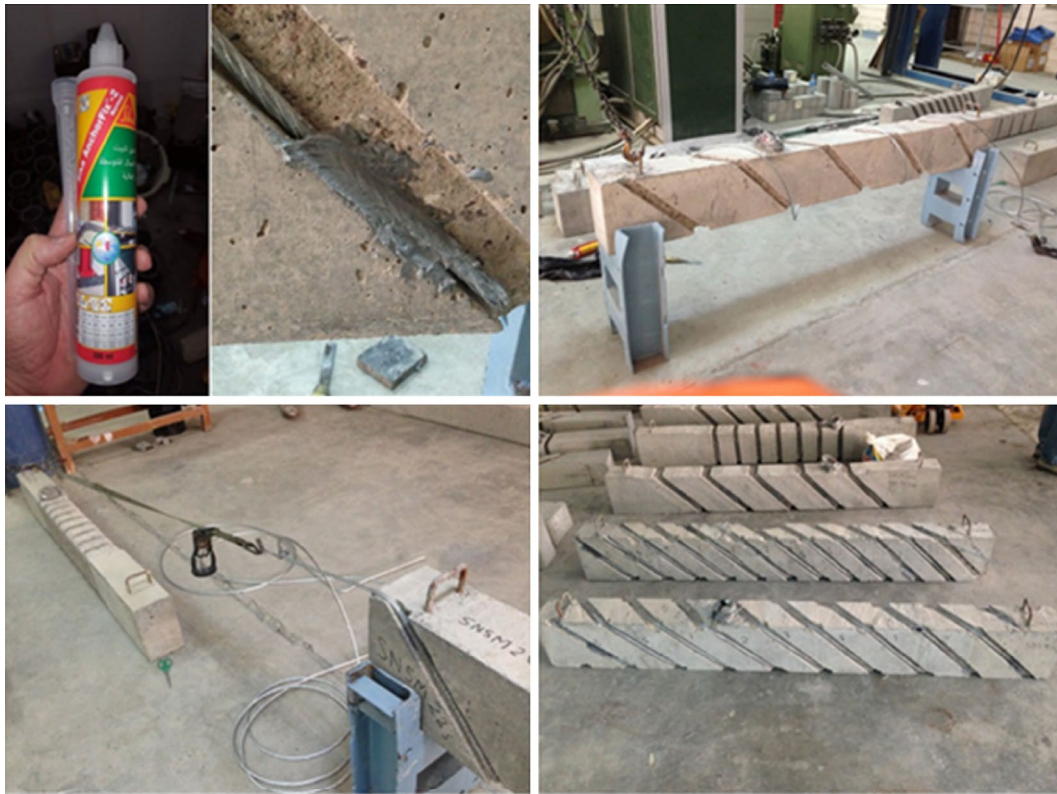
Fig. 4 Continuous spiral NSM steel wire rope installation.
