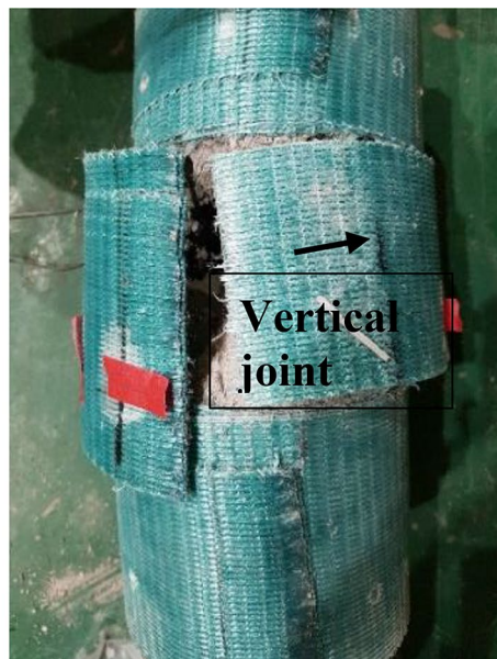
b C-P2-50mm: debonding and rupture
