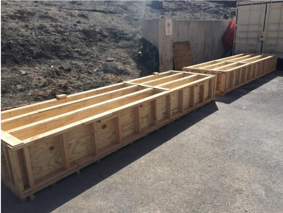
Figure 3-11: Formwork Platforms for Twelve Concrete Beam (wall bracing not shown for clarity).
