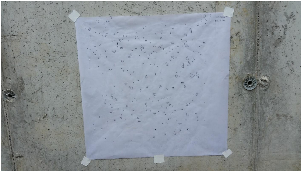
Fig. 6.14 Cast-in-place wall being measured by NJIT student researchers on active construction site
