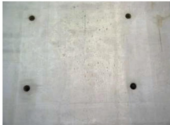
(a) Close view perpendicular to wall (tie holes as specified)
