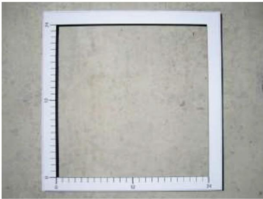
Fig. 3.2a(b)—Close-up view of wall Fig. 3.2a(a) with 24 x 24 in. (610 x 610 mm) measuring frame.
