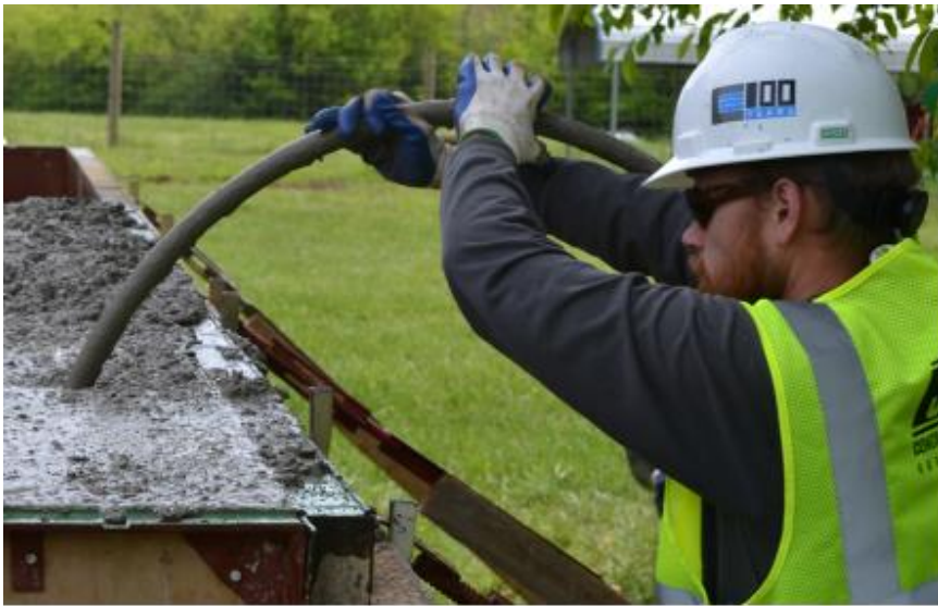
Photo 6. Vibration with a 2-in.-diameter internal vibrator
