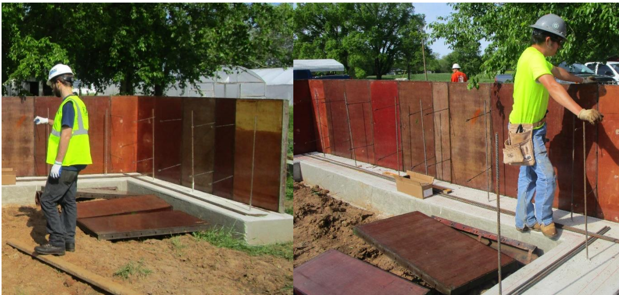
Photo 2. N and W outside wall forms
