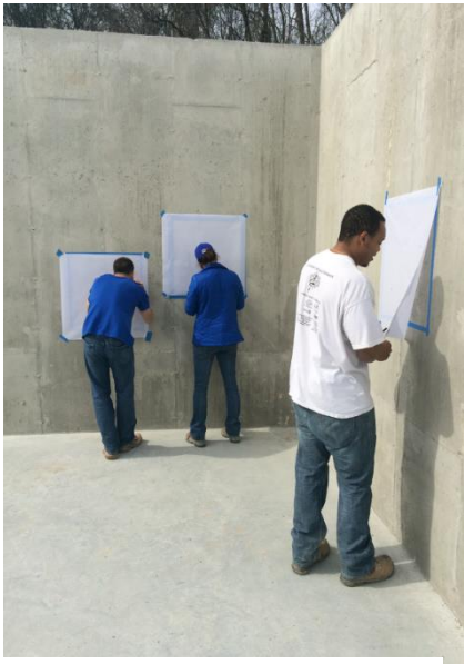
Large residence wall
