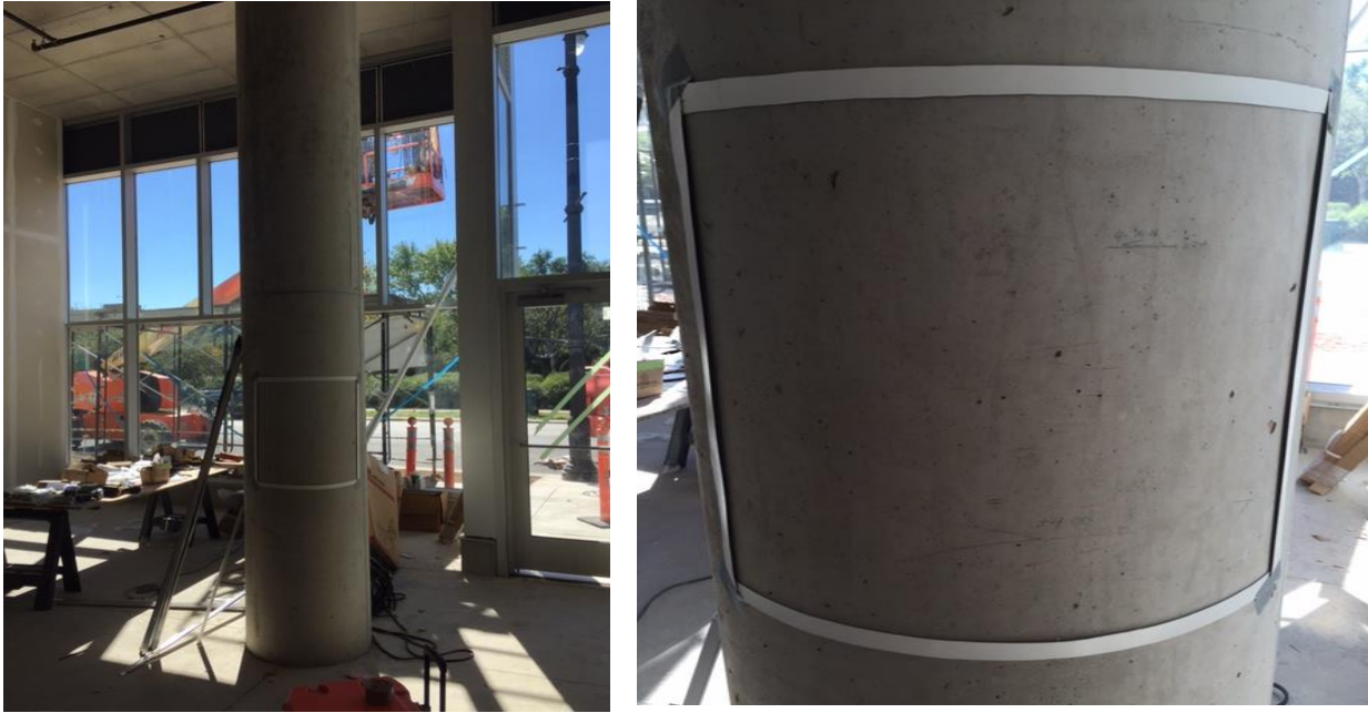
Fig. 6.19 Lab B circular column viewed from 20 ft and close-up of the sampled area. SVR for one sample = 0.4%.
