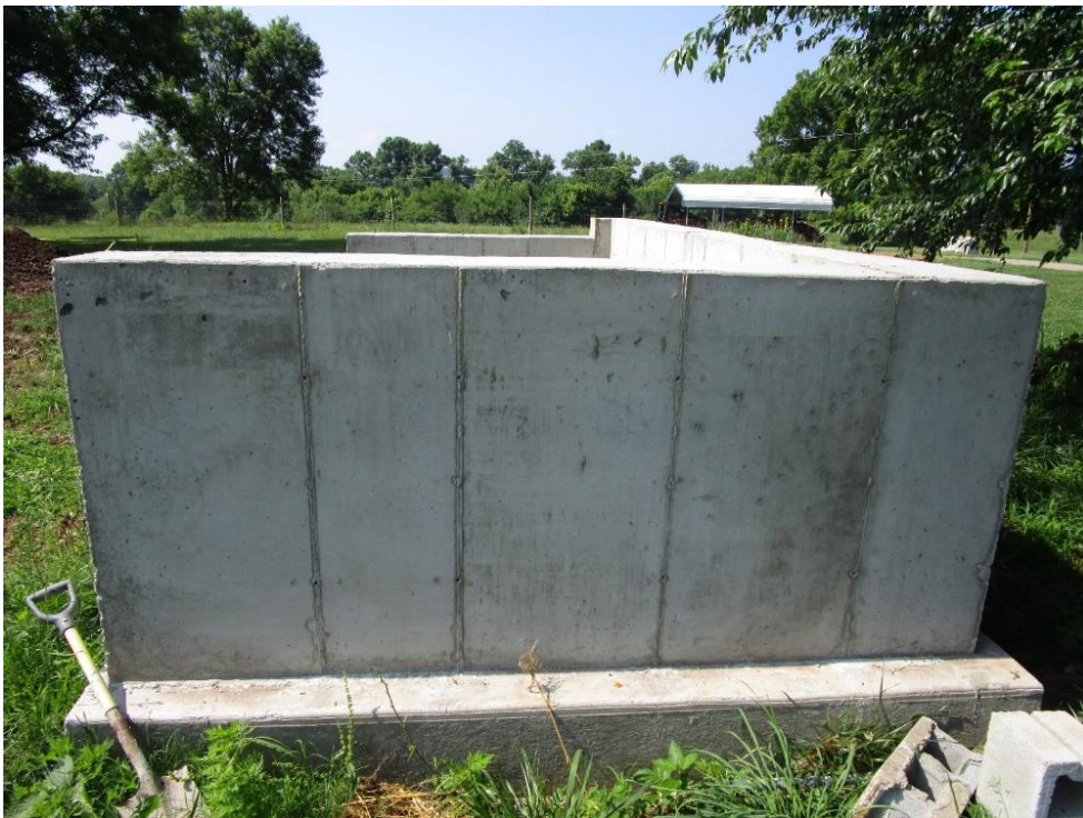
Photo 8 Outside face, north wall 6 weeks after forms were stripped. Note that much but not all of the discoloration is less apparent.
