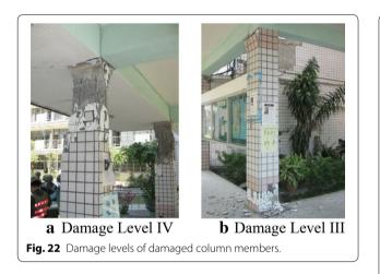
(Fig. 22a). Additionally, Fig. 22b shows a column with flaking tile and brick, which was classified as damage level III.
