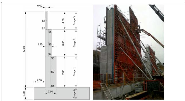
Fig. 15 Retaining wall construction in Loja (Granada, Spain): a main dimensions of the wall in meters, location of the temperature sensors S1 to S8 and indication of the construction stages and, b in situ construction of the wall.
