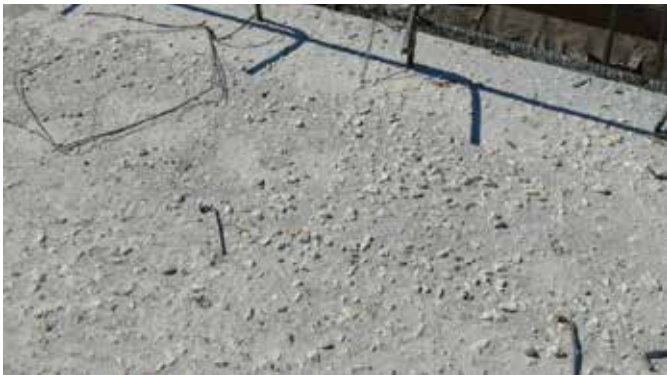
Fig. 1: An intense rainstorm can cause excessive loss of surface paste
