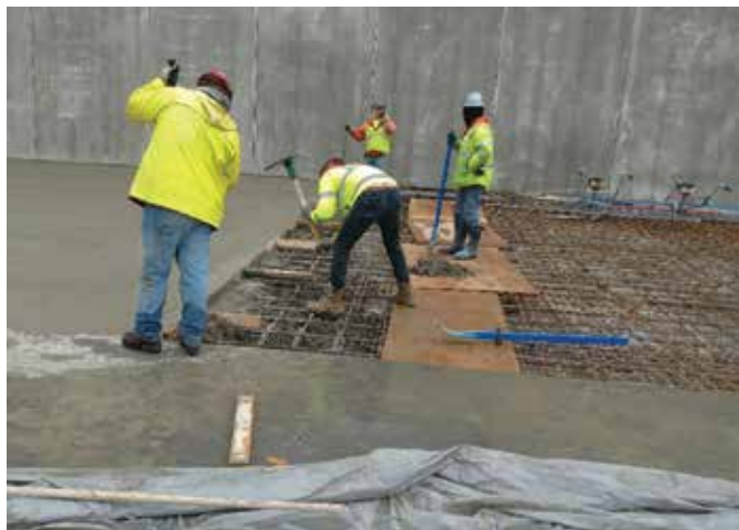
Fig. 5: Installation of an emergency bulkhead
