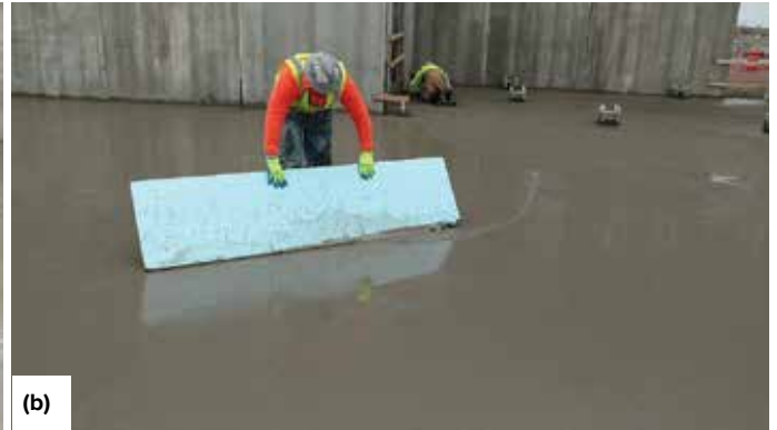
Fig. 6: Removal of rainwater from concrete surface: (a) using a squeegee and hose; and (b) using a foam insulation board
