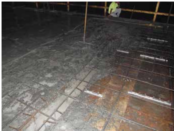
Fig. 4: Freshly placed concrete with rainwater puddles
