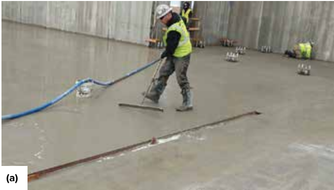
Fig. 6: Removal of rainwater from concrete surface: (a) using a squeegee and hose; and (b) using a foam insulation board
