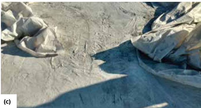
Fig. 2: Examples of concrete exposed to rainwater after it has been placed and floated: (a) a weakened surface; (b) shallow depth of the weakened surface; (c) surface marring caused by a protective cover; and (d) pockmarks caused by rain droplets
