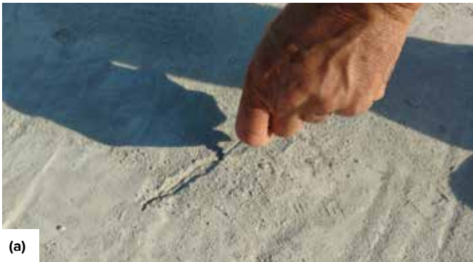
Fig. 1: An intense rainstorm can cause excessive loss of surface paste
