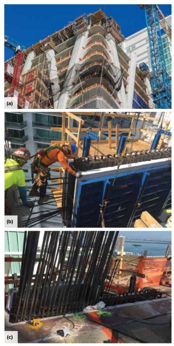
Fig. 5: The shape of the building from level 10 to 32 includes large balconies: (a) the balconies are supported by arch-shaped column brackets (*photo courtesy of ODP Architects*); (b) the brackets were constructed using GFRC forms that were assembled around reinforcing cages (*photo courtesy of Plaza Construction*); and (c) the brackets were anchored to the columns (*photo courtesy of Plaza Construction*)
