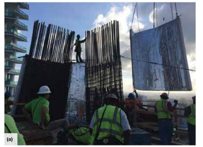
Fig. 3: GFRC forms were assembled around the reinforcing bar cages and clamped together: (a) the exterior forms included a vapor retarder (photo courtesy of Plaza Construction); and (b) steel frames and nylon straps were used to confine cast-in-place concrete (photo courtesy of ODP Architects)
