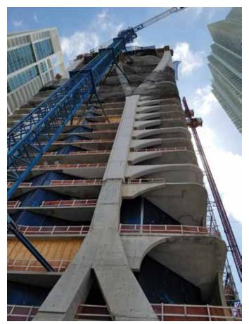
Fig. 2: While traditional removable wood formwork was used to construct the columns and brackets for the lower floors, stay-in-place GFRC formwork units were used to construct the columns and brackets above the 14th floor. Elevated slabs were cast on conventional flying tables (photo courtesy of ODP Architects)
