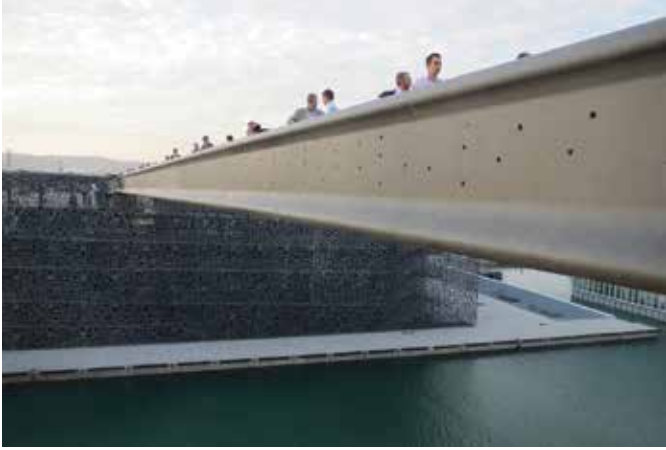
Post-tensioned UHPC channel girder in the MuCEM pedestrian bridge, Marseille, France (photo courtesy of Ben Graybeal)
