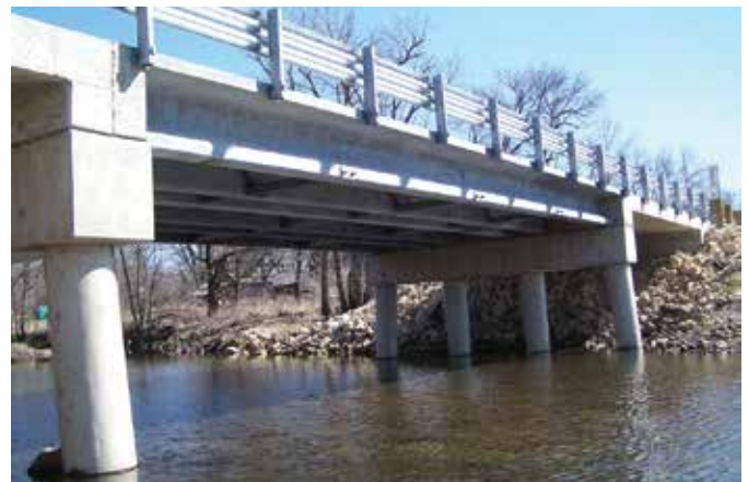
UHPC pi-girder bridge, Buchanan County, IA (photo courtesy of Ben Graybeal)
