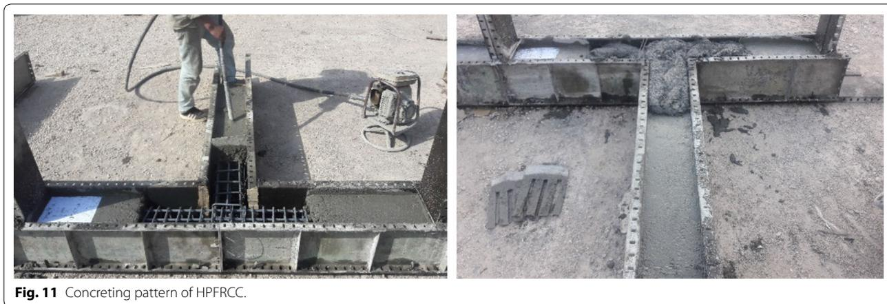
Fig. 11 Concreting pattern of HPFRCC.
