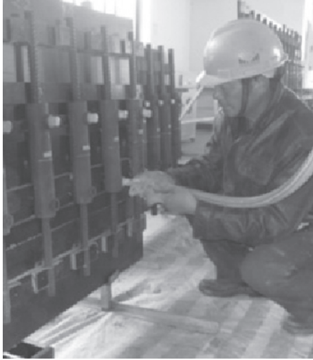
Fig. 2 Pouring grout in splice specimens.
