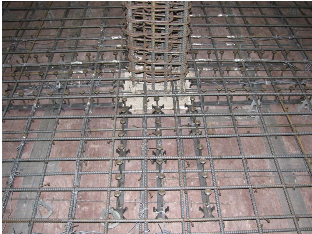
Figure 1-2: Orthogonal Stud Rail Arrangement
