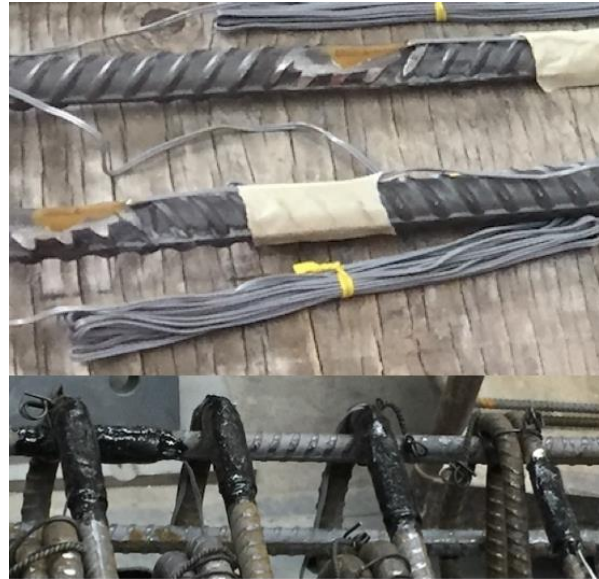
Figure 2.16: Strain Gauge Installation (Top) and Strain Gauges with Finished Coatings (Bottom)
