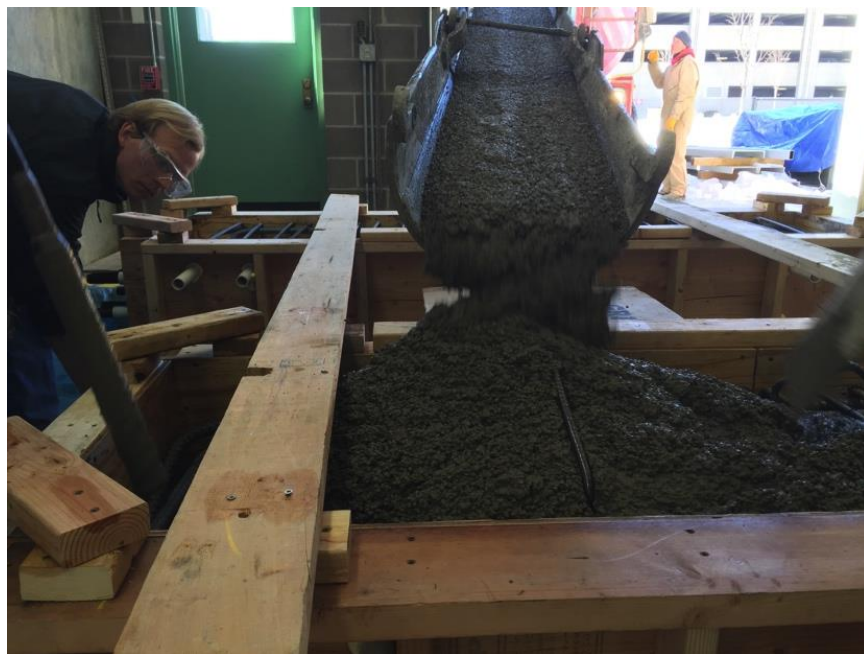
Figure 2.10: End Blocks Being Cast
