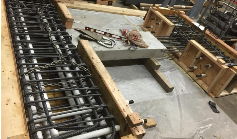
Figure 2.9: Precast FRC Coupling Beam Being Inserted Into End Block Reinforcement and Forms
