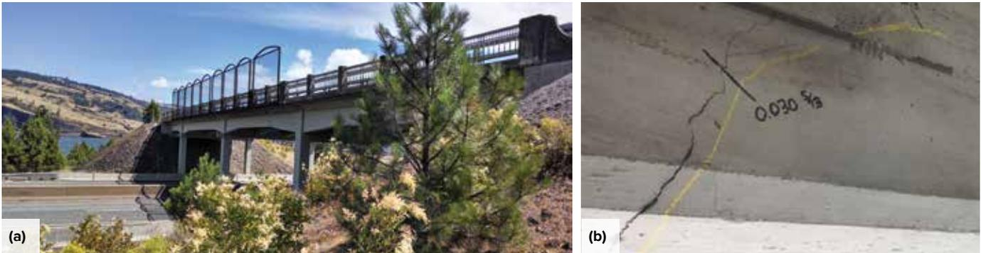
**Fig. 2:** The Mosier bridge is an overpass for a secondary road crossing I-84 in Oregon: (a) overall view of structure; and (b) cracks were observed near cutoff points for flexural reinforcement (photos courtesy of ODOT)
