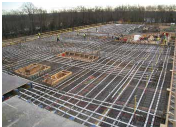
Fig. 2: Workers place PT tendons in a floor slab
