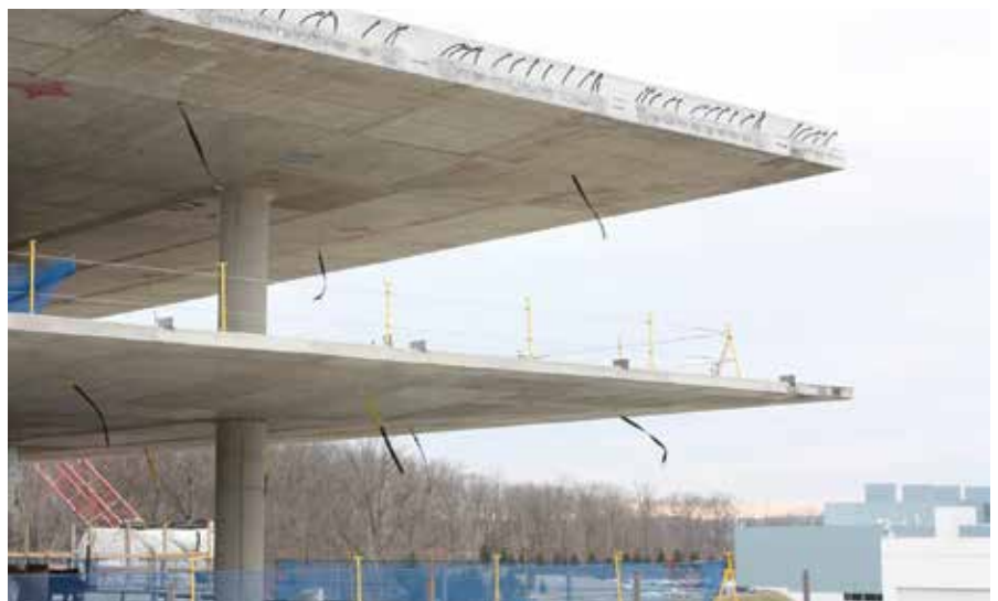
Fig. 5: View of 40 ft (12 m) cantilever at corners
